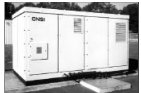
Figure 6. ONSI's Commercial PAFC PC25 200kWe Cogeneration Power Plant System
