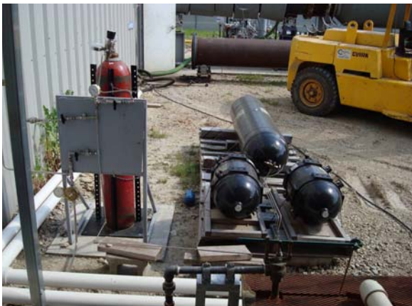
Figure 3: Manifold and Tanks Used to Blend Fuel.
