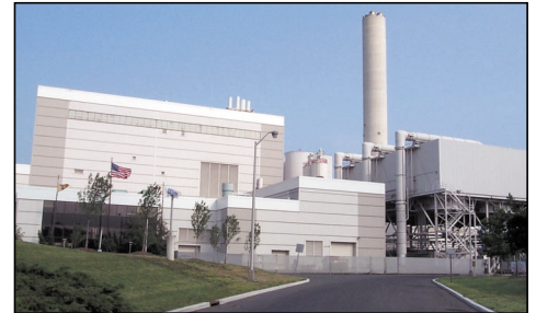
Union County Resources Recovery Facility in Rahway, N.J.
