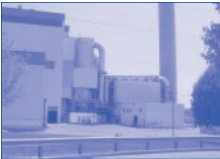
Tour of Montanay Montgomery County Waste To Energy Facility
