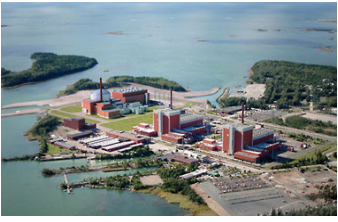
The 1,600 megawatt nuclear power plant is under construction at a place called Olkiluoto, Finland.
