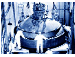
Men working on a reactor head
