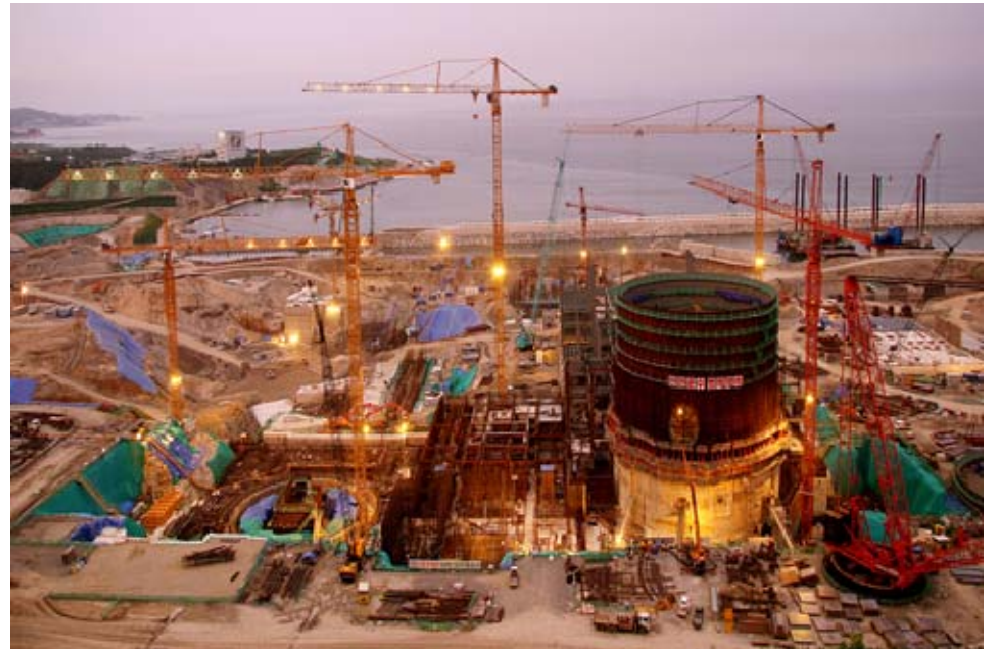
Shin-Kori 1&2 under construction in 2007
