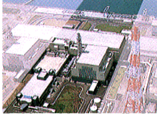
Kashiwazaki-Kariwa Nuclear Power Station Unit NO.6 of The Tokyo Electric Power Co., Inc.
