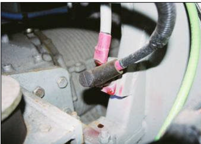
Photo 8b: Bulkhead Connection Bosch T1
